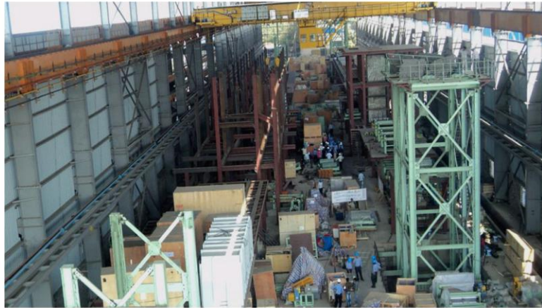
Colour coating line at Vasind
