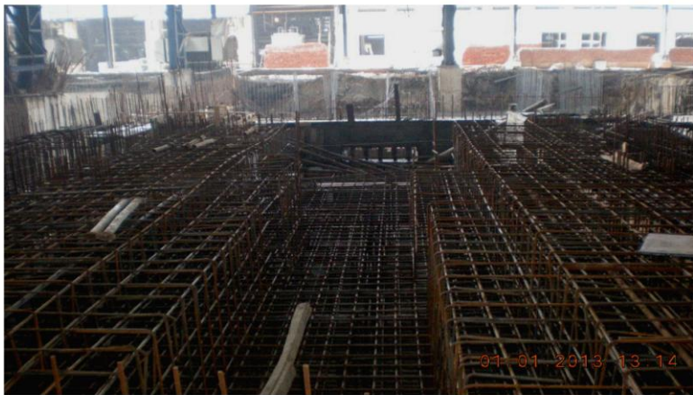
New Galvanizing line at Tarapur
